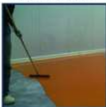
SISTEM EPOXIDIC AUTONIVELANT
